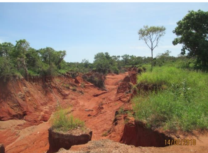
Erosion of a stormwater drain near Cable Beach following extensive water infiltration
