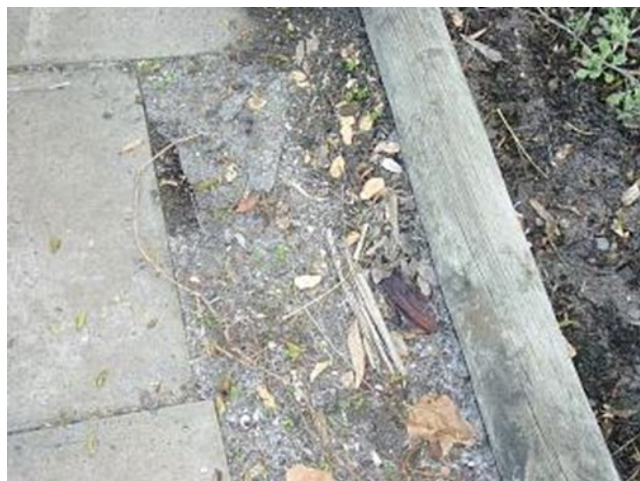
Images: Asbestos contamination from high-pressure water cleaning an asbestos roof
